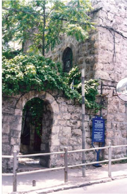
Fig. 5. The entrance to the building of the hospital.
